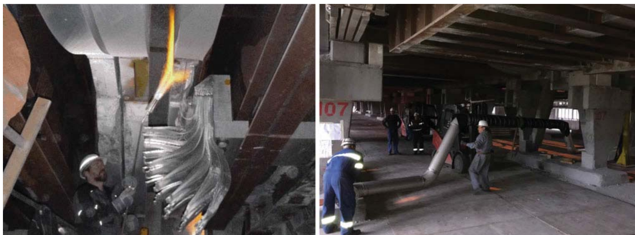
Fig. 7 Basement activities implementing piping for the shell heat exchangers
